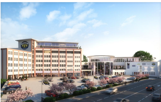
3-Glocken-Center in Weinheim
